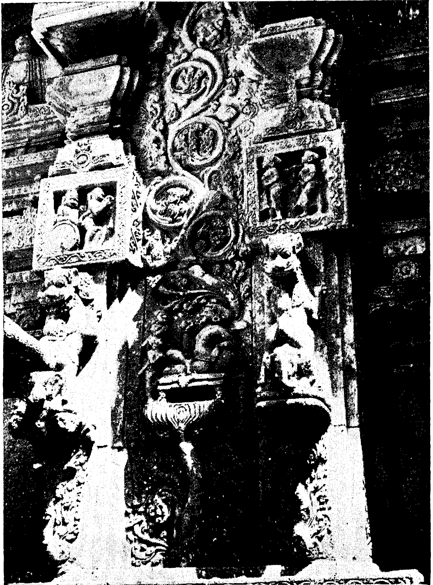
Fig. 10: The Outer Wall of the Central Shrine
